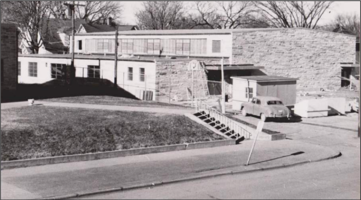
Construction of Cleary Hall - 1963
